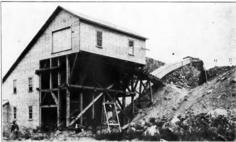
Primary Crusher House and Belt Conveyor to Secondary Crusher
